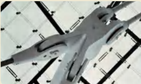
Nodal points of suspended roof construction of the Olympic Stadium in Munich, Germany
